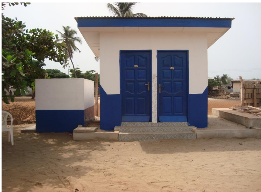
Figure 8: WC Toilet facility constructed by Anlo Afiadenyigba WSDB
