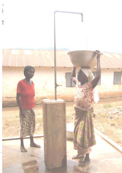
Figure 4: Standpipe in the Volta Region of Ghana
