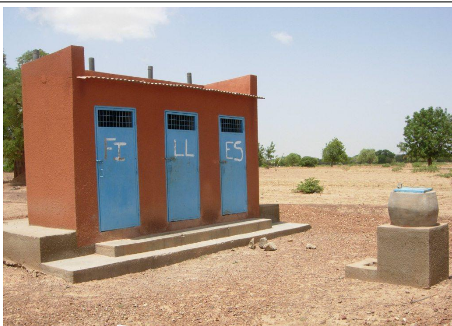
Picture 1: Separate latrine block for girls with a handwashing facility close by (Burkina Faso)
