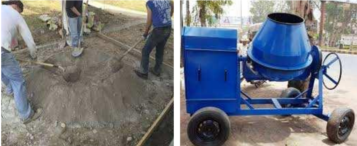
Fig-22: Hand and mechanical mix
