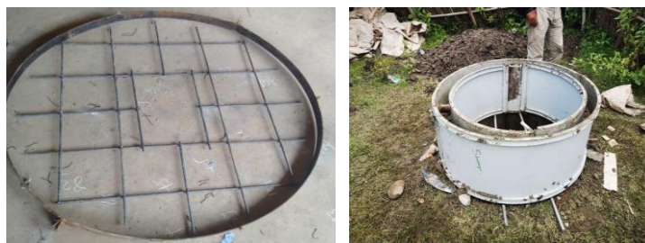
Fig.14: Steel form work/ mold
