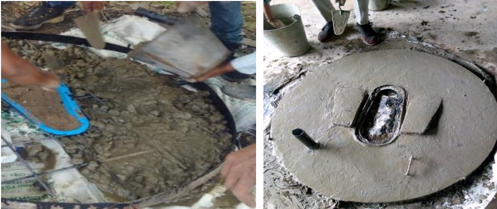
Fig. 25: Placing of concrete.
