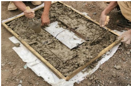
Fig-26: Hand and mechanical compaction
