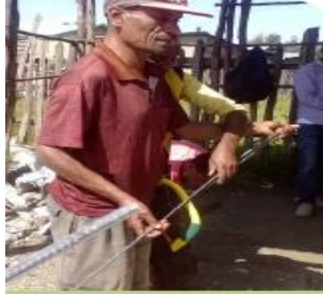
Fig-7: Cutting of rebar.
