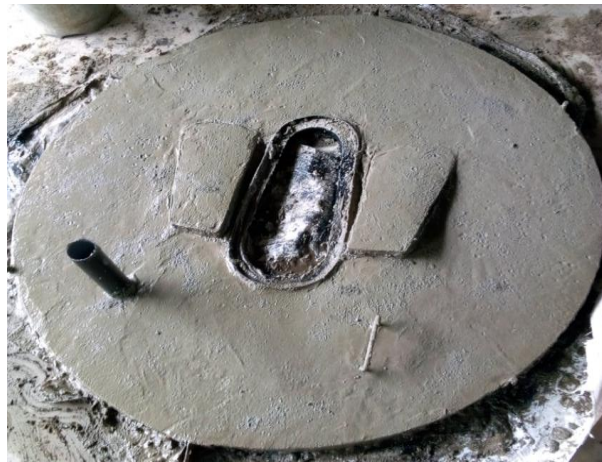
Fig. 29 circular concrete slab
