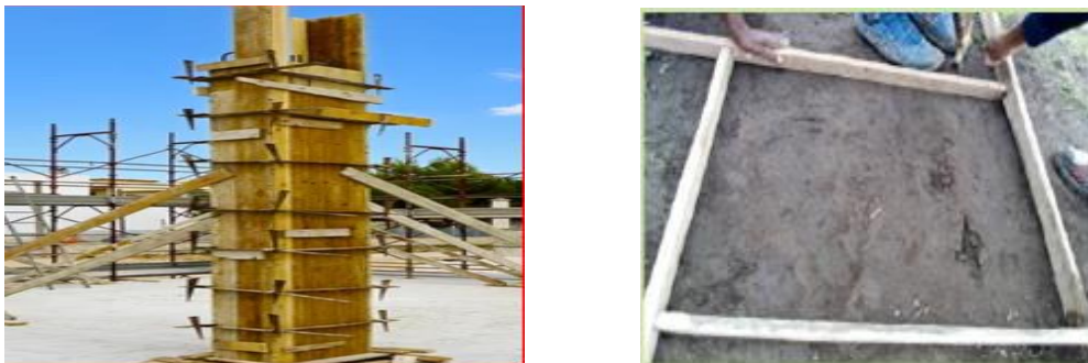
Fig-12: Form work to cast slabs and column
