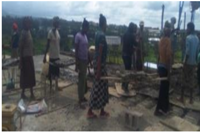
Fig. 23: Transporting of concrete.
