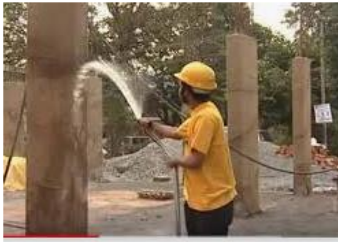
Fig. 28- Curing of concrete
