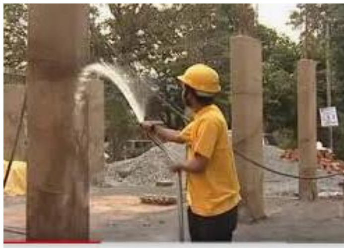
Fig. 28- Curing of concrete
