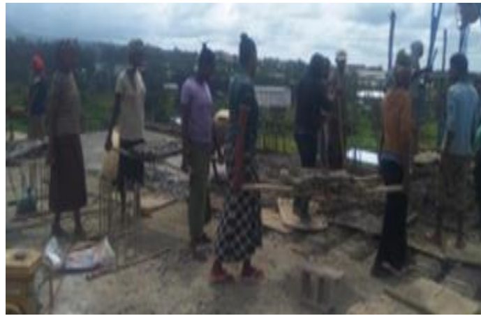
Fig. 23: Transporting of concrete.
