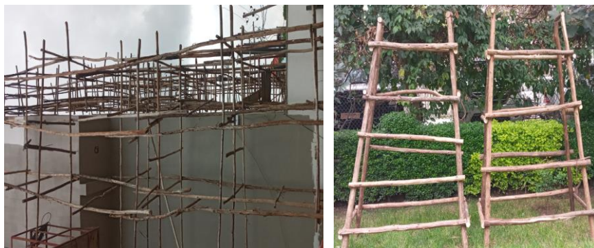
Fig. 15: Wooden scaffolding
