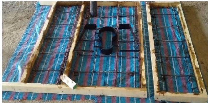
Fig. 13: Wooden form work to cast concrete slab
