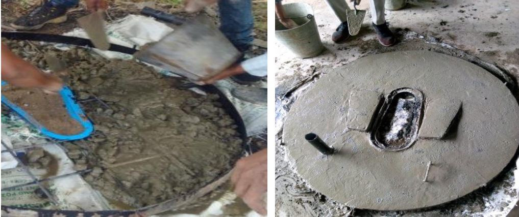
Fig. 25: Placing of concrete.
