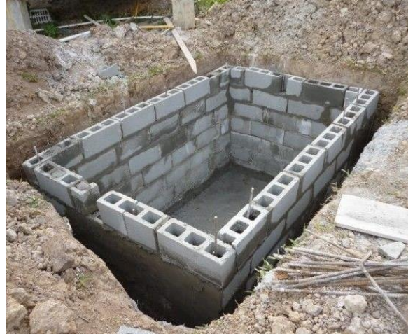
Figure.3.19. Erecting rectangular wall
