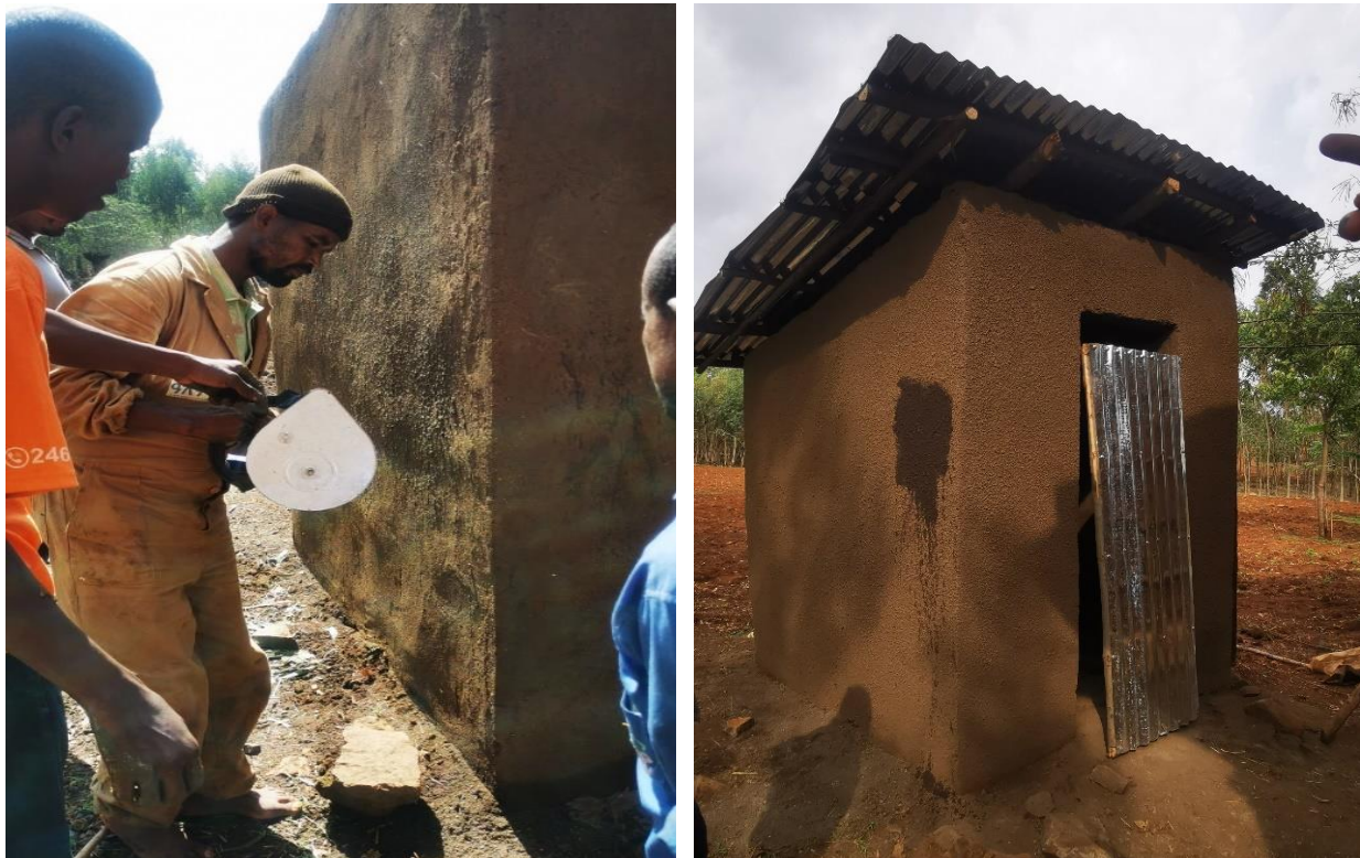
Figure: 2.3. Plastering of toilet mud wall with cement mortar
