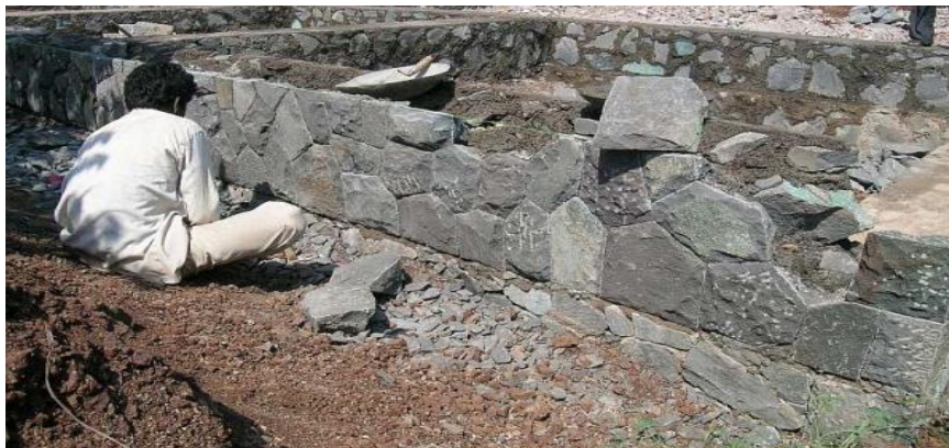
Figure.3.6 Sample of masonry work
