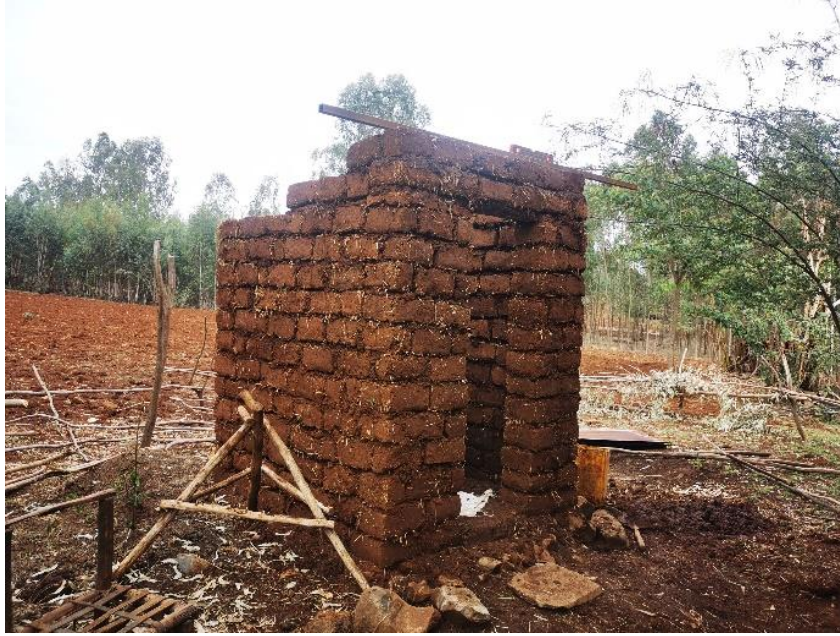
Figure: 2.2. Toilet wall construction with mud block
