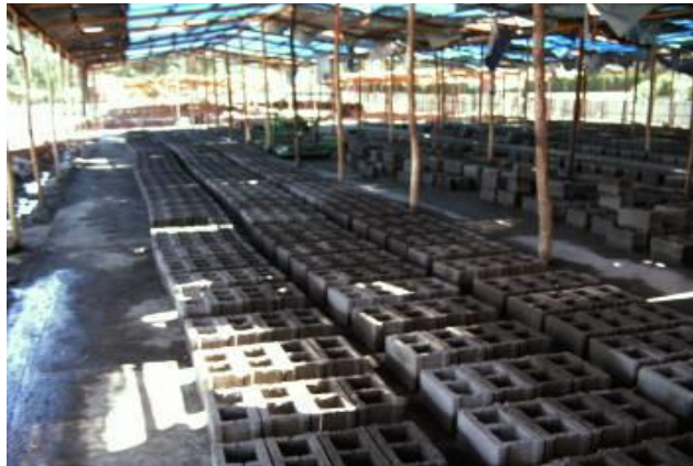
Figure-1.10. Shade for Freshly Cast Block Protection....
