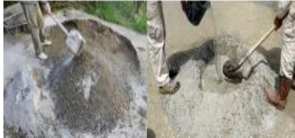
Figure.1.1. Hand mixing
