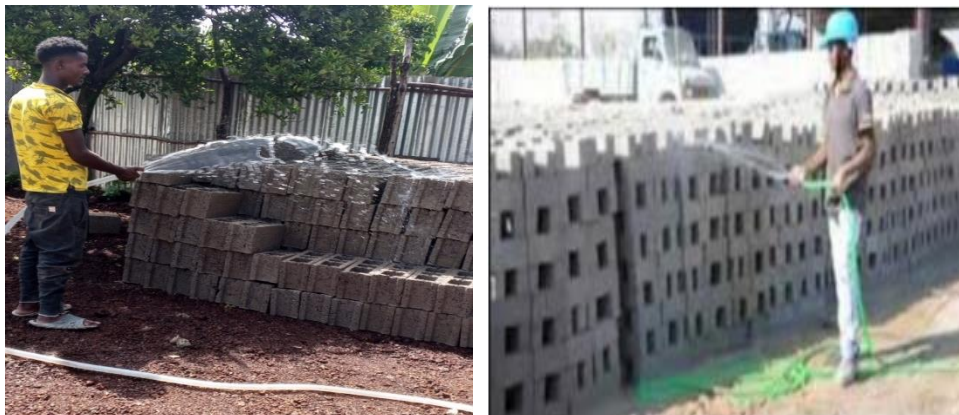
Figure: 1.11. Curing of concrete block
