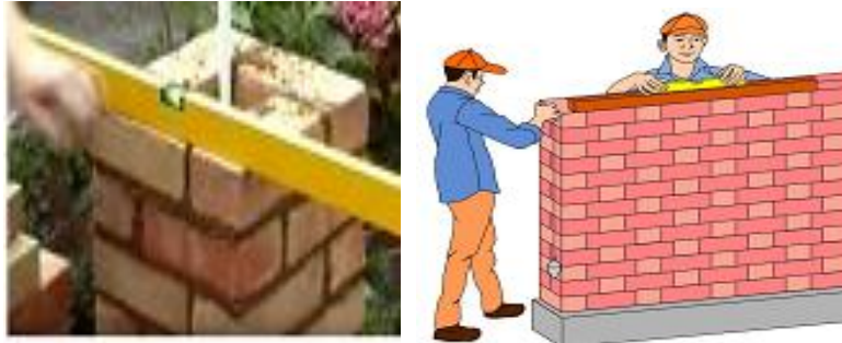
Figure-3.16: checing horizontal alignment with sprit level
