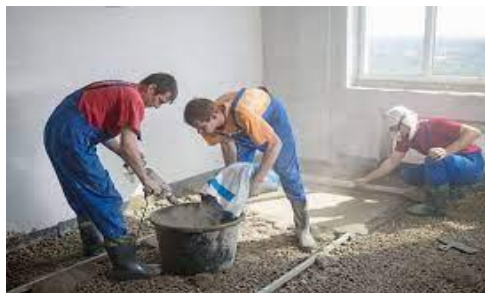
Figure: 4.4. Divide up your floor area & placing the floor screed mixture
