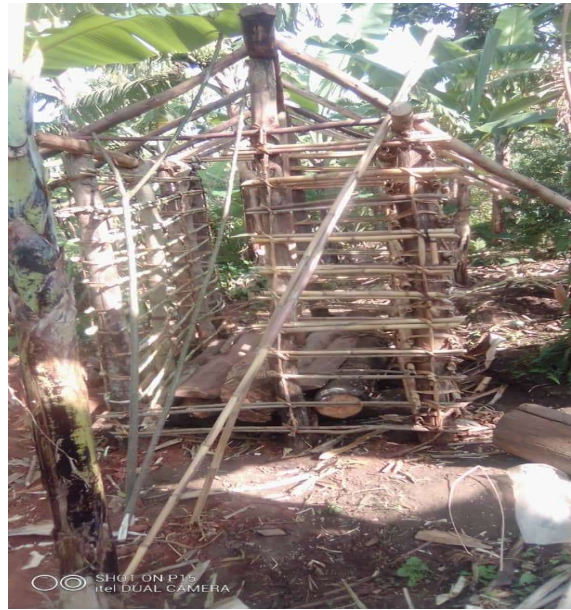
A latrine under construction in Nyakasojo Village in Mugusu S/C
