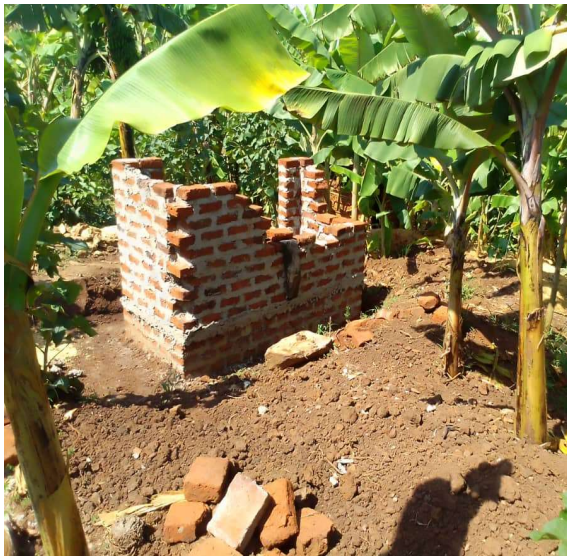
An improved pit latrine under construction in Kyantambara zone, Kasenda.
