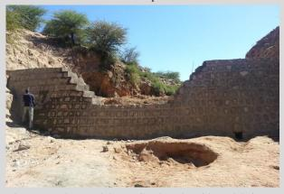
Almost complete sand dam at Gende Roba with work being completed on the front wall. Sand dams are constructed aboveground and fill with new sediment creating a deeper sand aquifer. The dam can be raised, capturing more sand and increasing the storage capacity.
