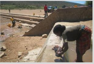
*Bishan-bahe* (where the water comes out) was reconstructed in 2010 by HCS after flood damage (it was built in 1993). There is a very wide sand dam with an infiltration gallery and canal to the irrigated fields. Hand dug wells and boreholes for domestic supply are recharged by the structure. The community need help from government/NGOs for even minor maintenance and the scheme potential is under-utilized.
