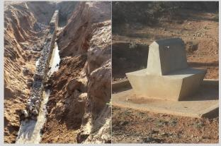
Reconstruction of a section of the sub-surface dam at Kenchera and a completed domestic water supply tapstand linked to the system (January 2014).
