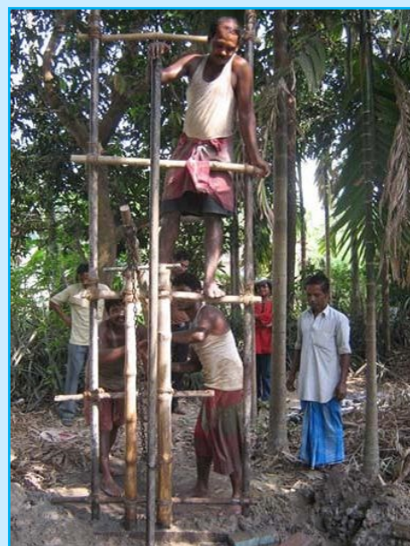
Rota-sludging in India
