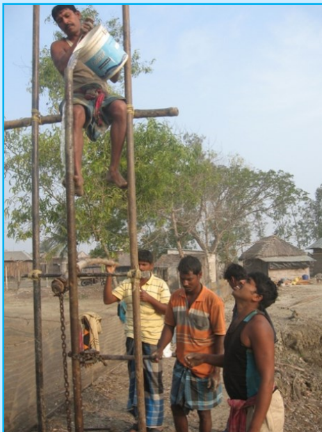
Rotary-sludge drilling in India
