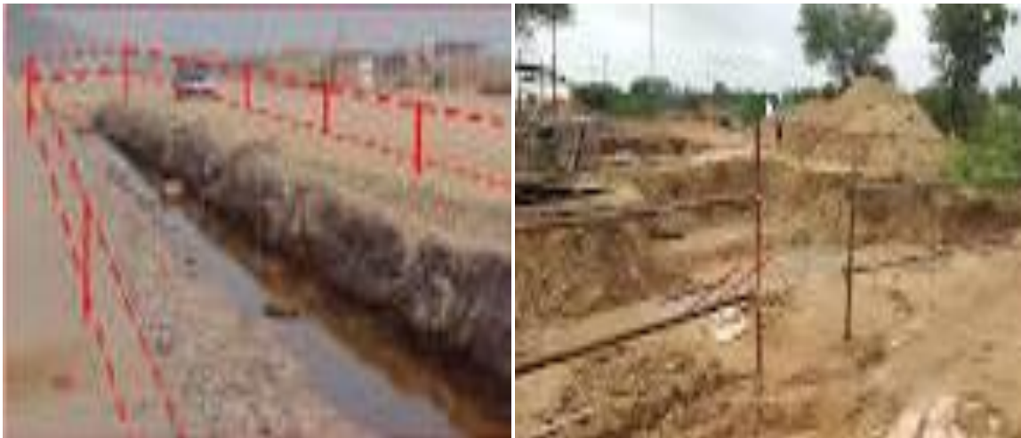
Figure-10: Barricade in excavation
