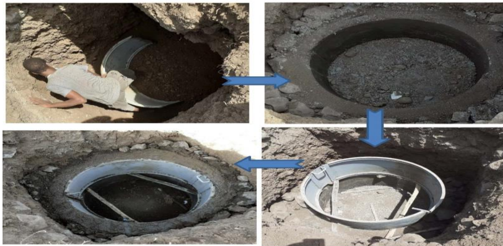
Figure-9: Cast on site inside pit.
