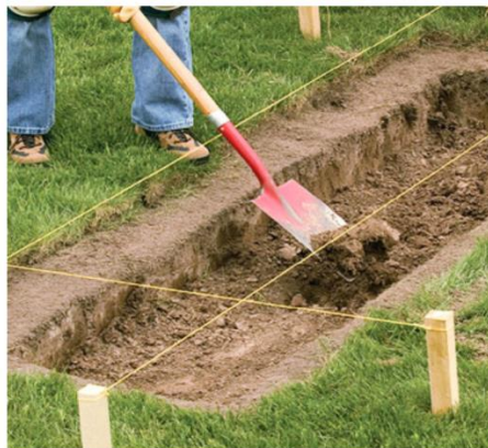
Figre-12: Trench excavation
