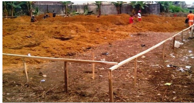
Figure-11: Excavation work
