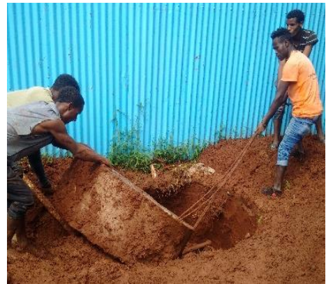
b). Precast concrete ring and transport to site
