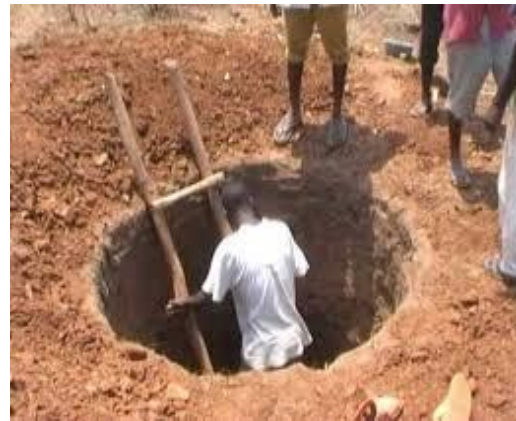
Fig-5: Circle latrine pit excavation
