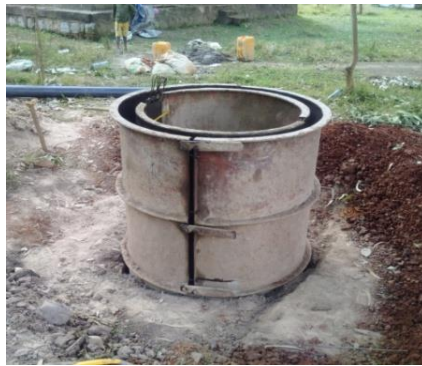
a) Concrete ring cast on pit
