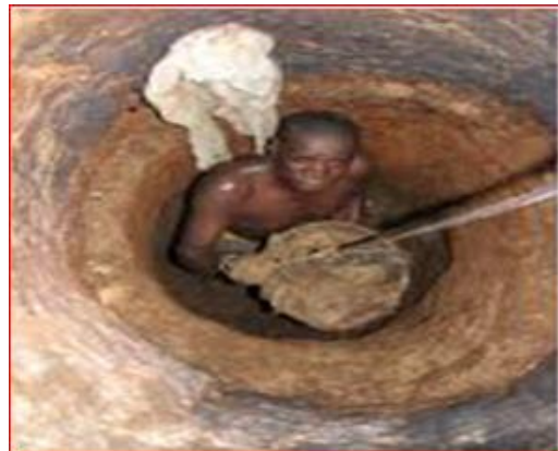
Figre-13: Circle trench excavation
