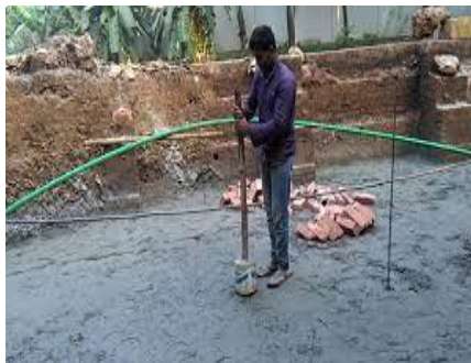
Fig-17: Manual Compaction
