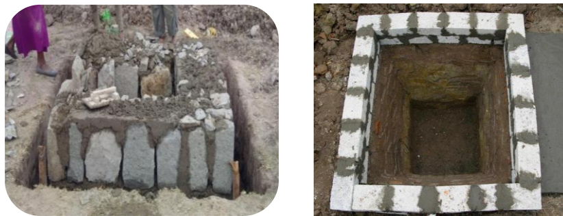
Fig-7: Under ground masonry wall construction
