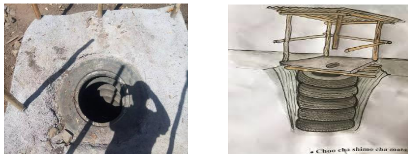
Fig-8: Used tyre pit lining.
