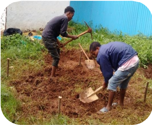
Fig-5: Circle latrine pit excavation
