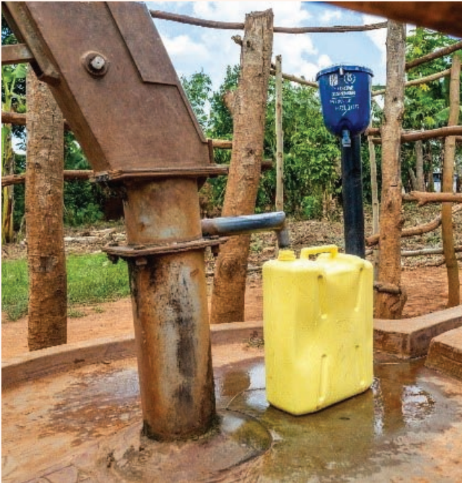
A chlorine dispenser installed by Evidence Action at a water point in Nakulyaku Village, Buwenge, Jinja. The chlorine dispenser is an easy to install device that sits beside the water source allowing those fetching water to release a pre-set 3 milliliters of chlorine, per 20 liters, into their freshly collected water. In 30 minutes, the water is safe to drink and, if well stored, will stay safe for up to three days.
