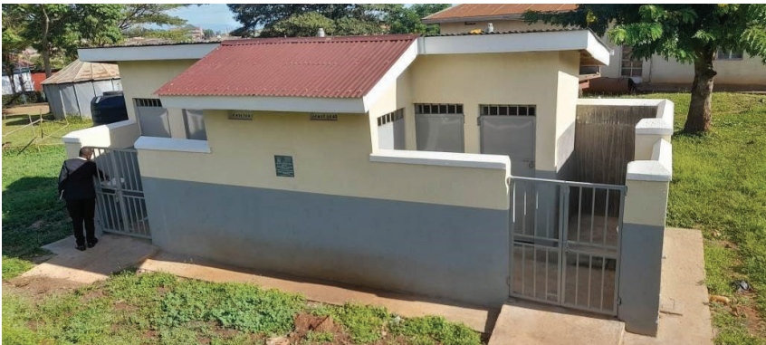
The new patient's sanitation facility at Rwiimi HCIII, Bunyangabu was commissioned in 2023. IRC photo.
