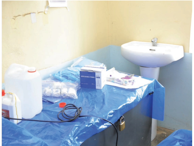
Services are safest for both health workers and patients when there is running water in the treatment rooms.
