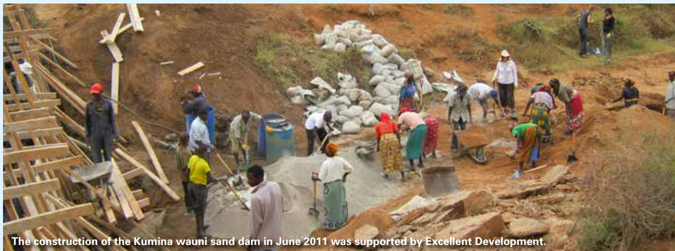
Community in Kenya passes rocks for building the Kumina wauni sand dam.
